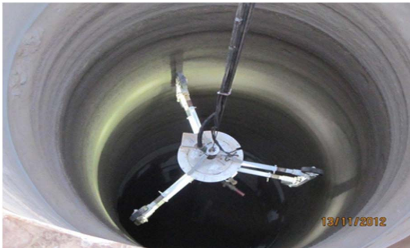
← Shotcreting vent shaft
