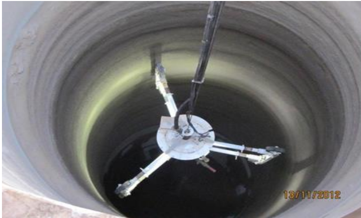
← Shotcreting vent shaft
