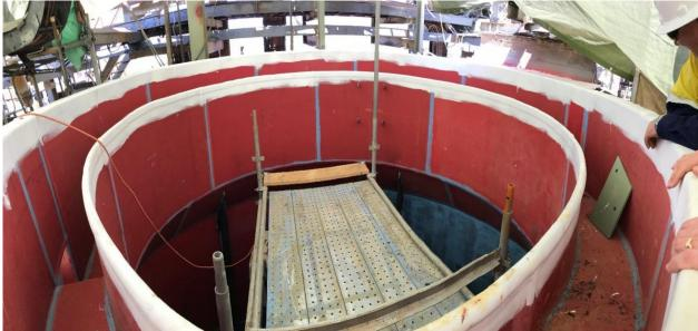
New rubber lining in the flotation cells
