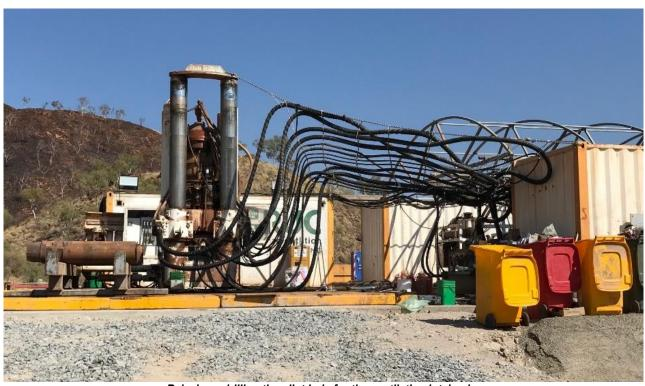
Raisebore drilling the pilot hole for the ventilation intake rise
