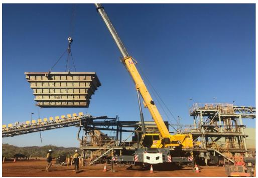
Re-installing the surge bin following installation of new liners
