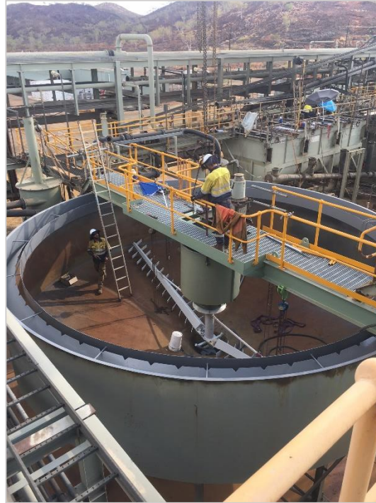
Refurbishment of tails thickener
