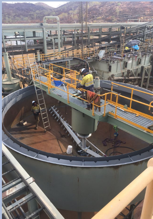
Refurbished concentrate thickener
