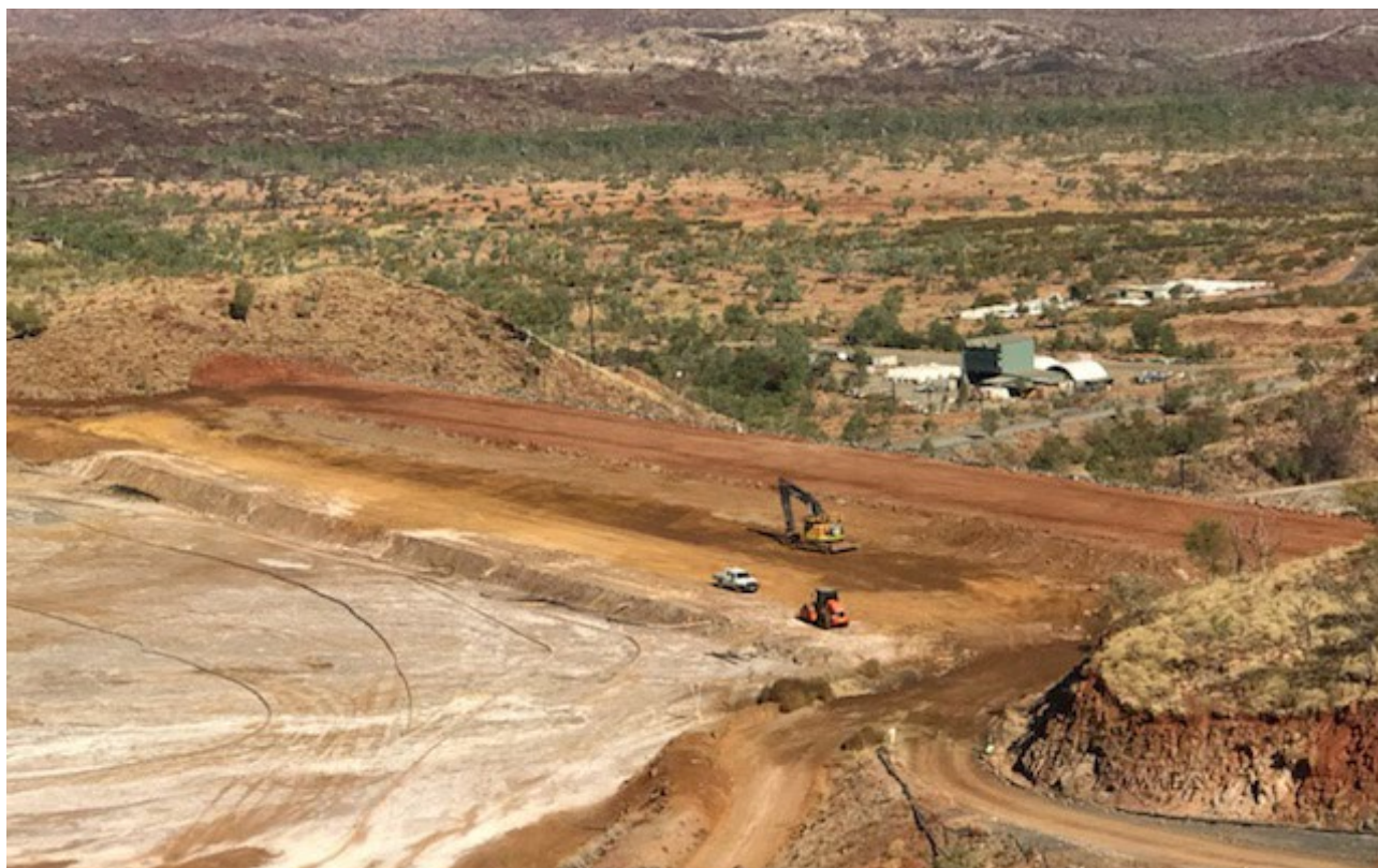
Tailings Storage Facility 3m wall lift
