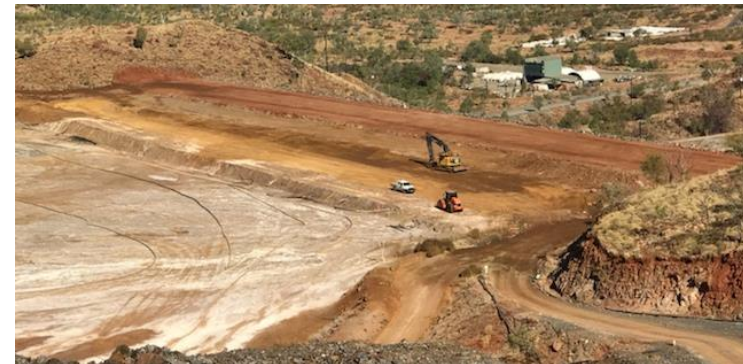
Tailings Storage Facility 3m wall lift
