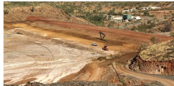
Tailings Storage Facility 3m wall lift
