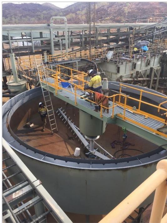
Refurbishment of tails thickener
