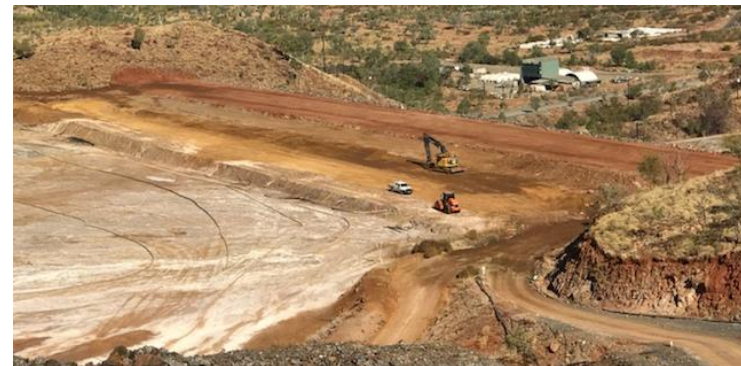
Tailings Storage Facility 3m wall lift
