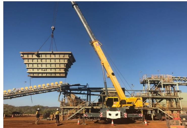
Re-installing the surge bin following installation of new liners
