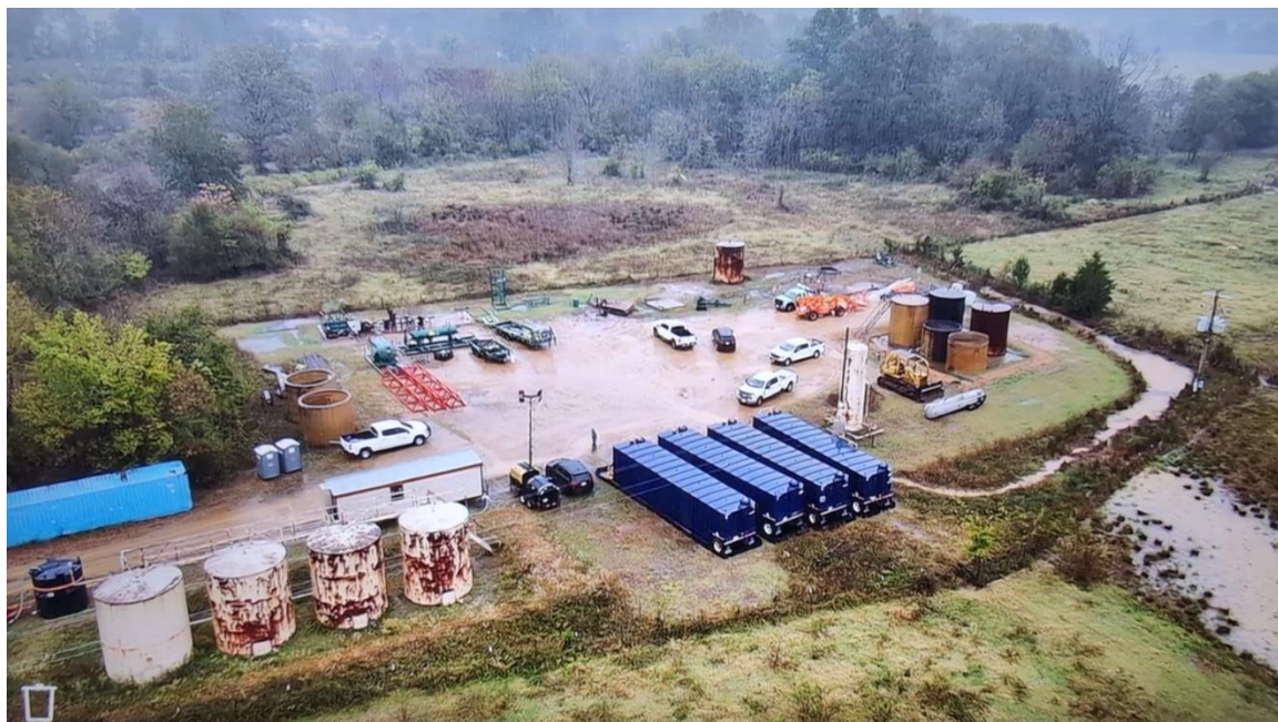
Figure 1. Pantera well location Lafayette County Arkansas.
