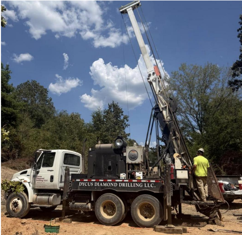
Figure 1. Dycus Rig on site at the first hole
