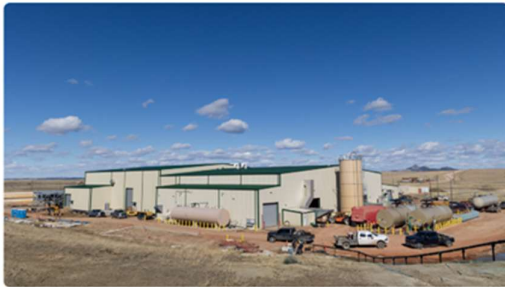
Central Processing Plant (Phase I & II)
