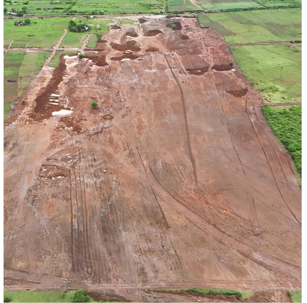
Bulk Earthworks – Process Plant Topsoil Removal
