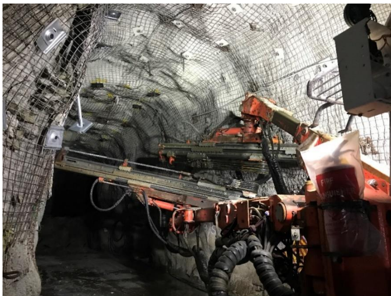
Photo 1: WestAuz drilling jumbo in the Golden Swan Drill Drive
