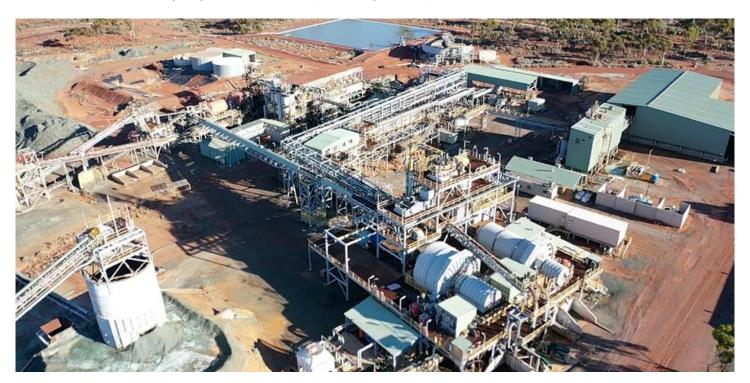
Figure 1 – Black Swan 2Mpta processing plant with the 150ktpa circuit located between the mills and float circuit
