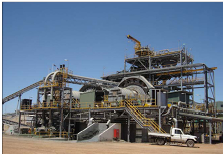
Figure 2: Black Swan Grinding Circuit (10MW of installed power)
