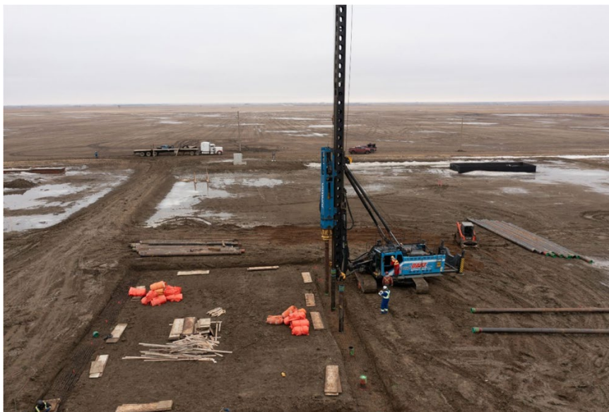
Figure 3: Installation of foundation piles at Pad#1
