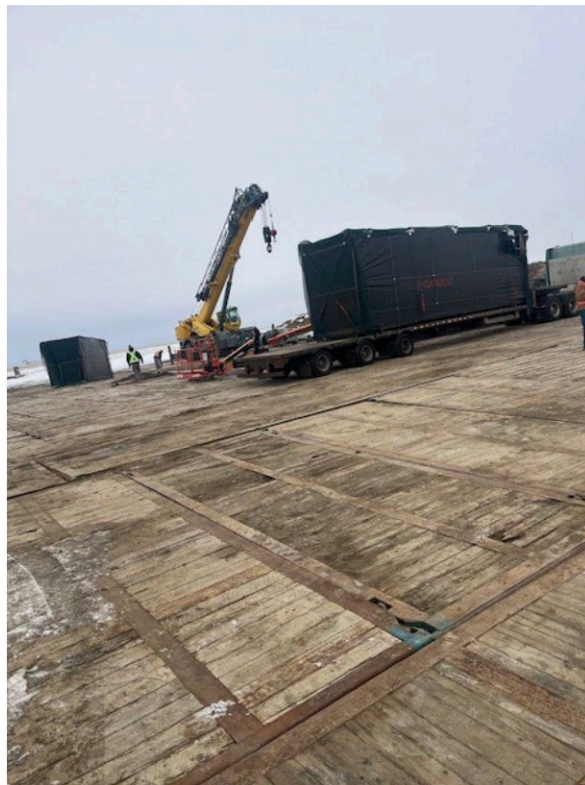
Figure 4: Building materials arriving on-site
