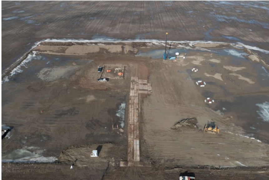
Figure 1: Aerial view of Pad #1 during foundation construction
