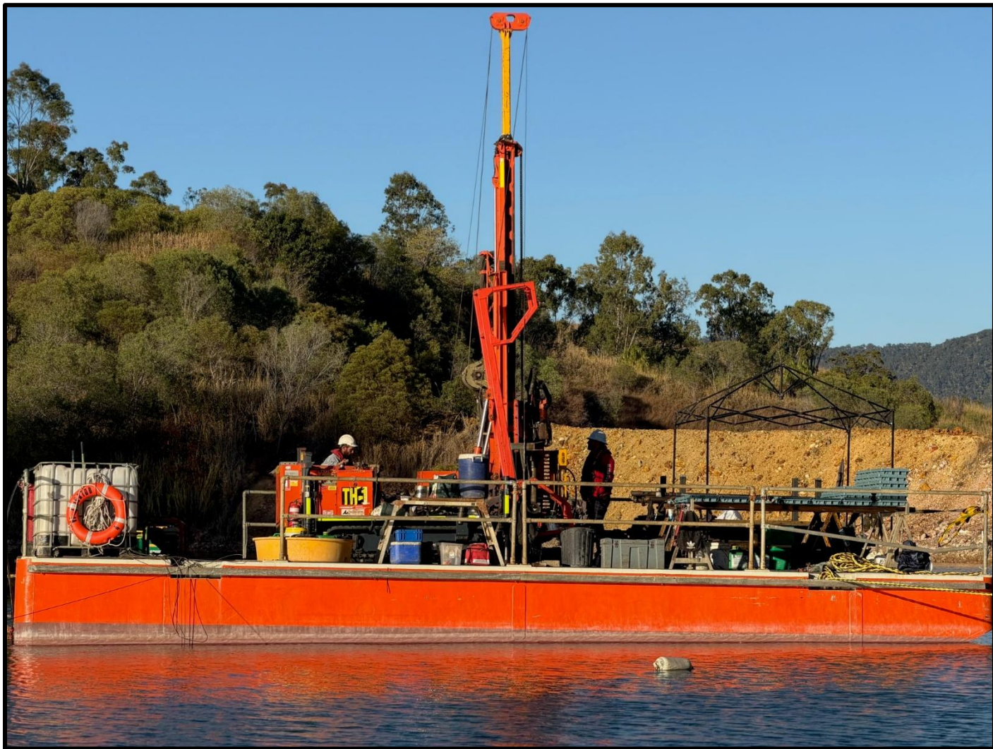
Figure 6 – Rig 19 Barge Drilling.
