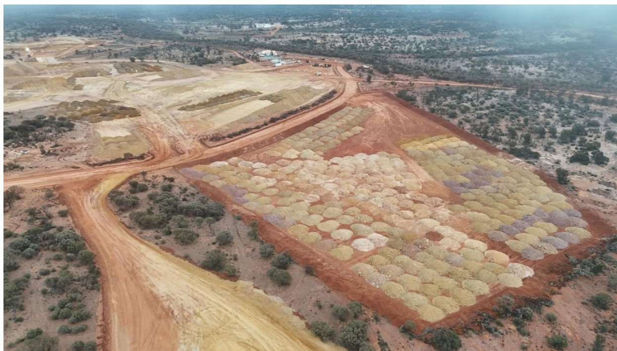
Figure 2: Ore stockpiling at the Redcastle Gold Project
