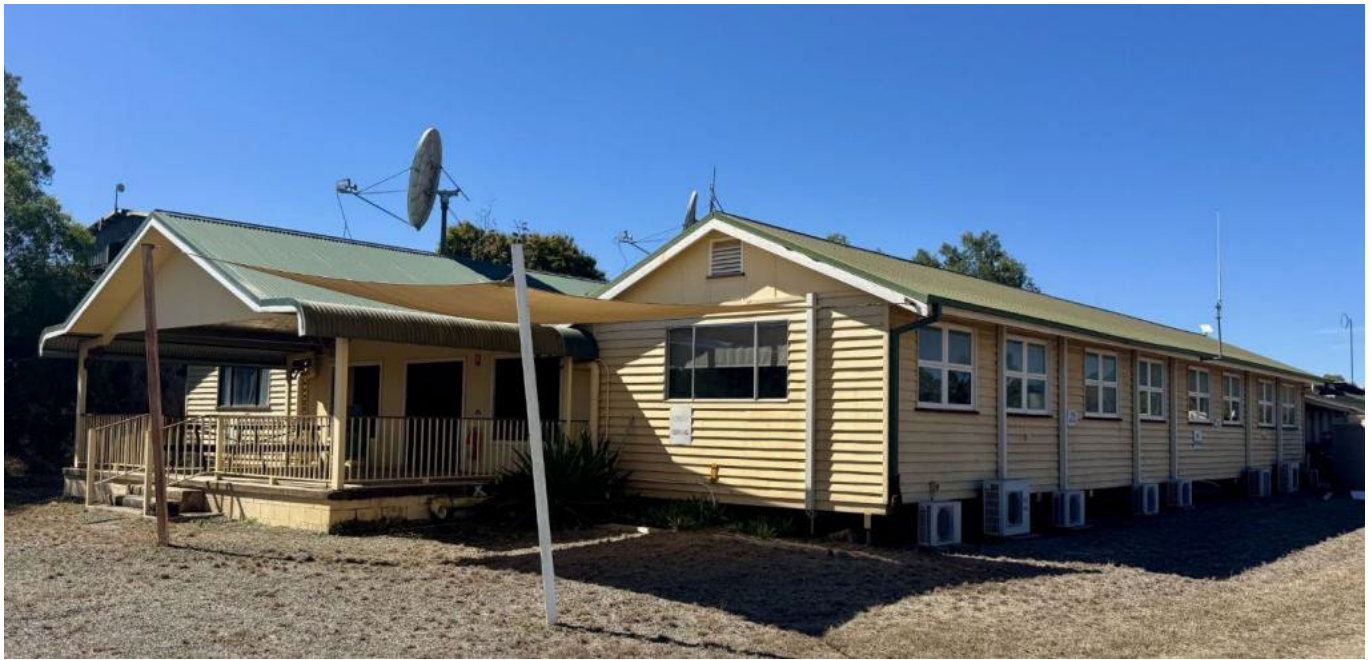
Figure 9 from ASX 8/9/26: Recommissioning of site office complex.
