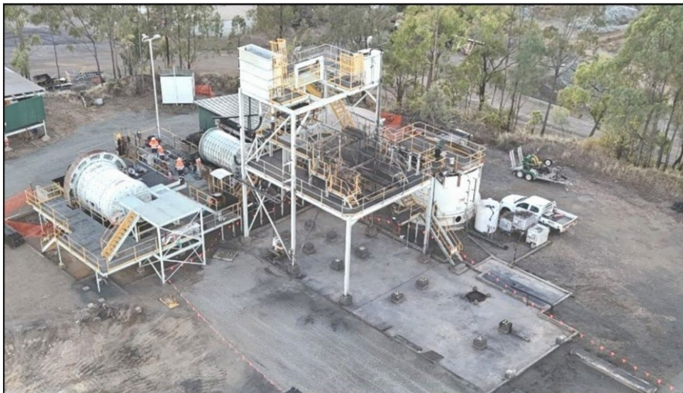
Figure 3 from ASX 8/9/26: Mt Moss Mill with all magnetite-related plant decommissioned on August 10, 2026. Ball mills have since been emptied, with liners stripped and lifted.
