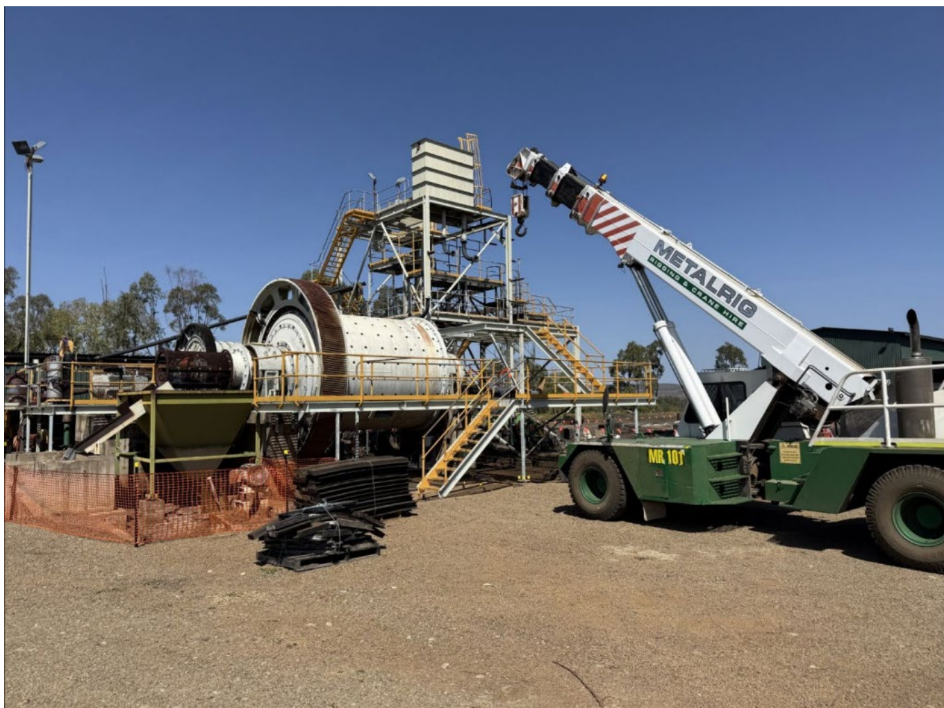
Figure 4 from ASX 8/9/26: Liners removed from ball mills and being craned out on 13 August 2026.
