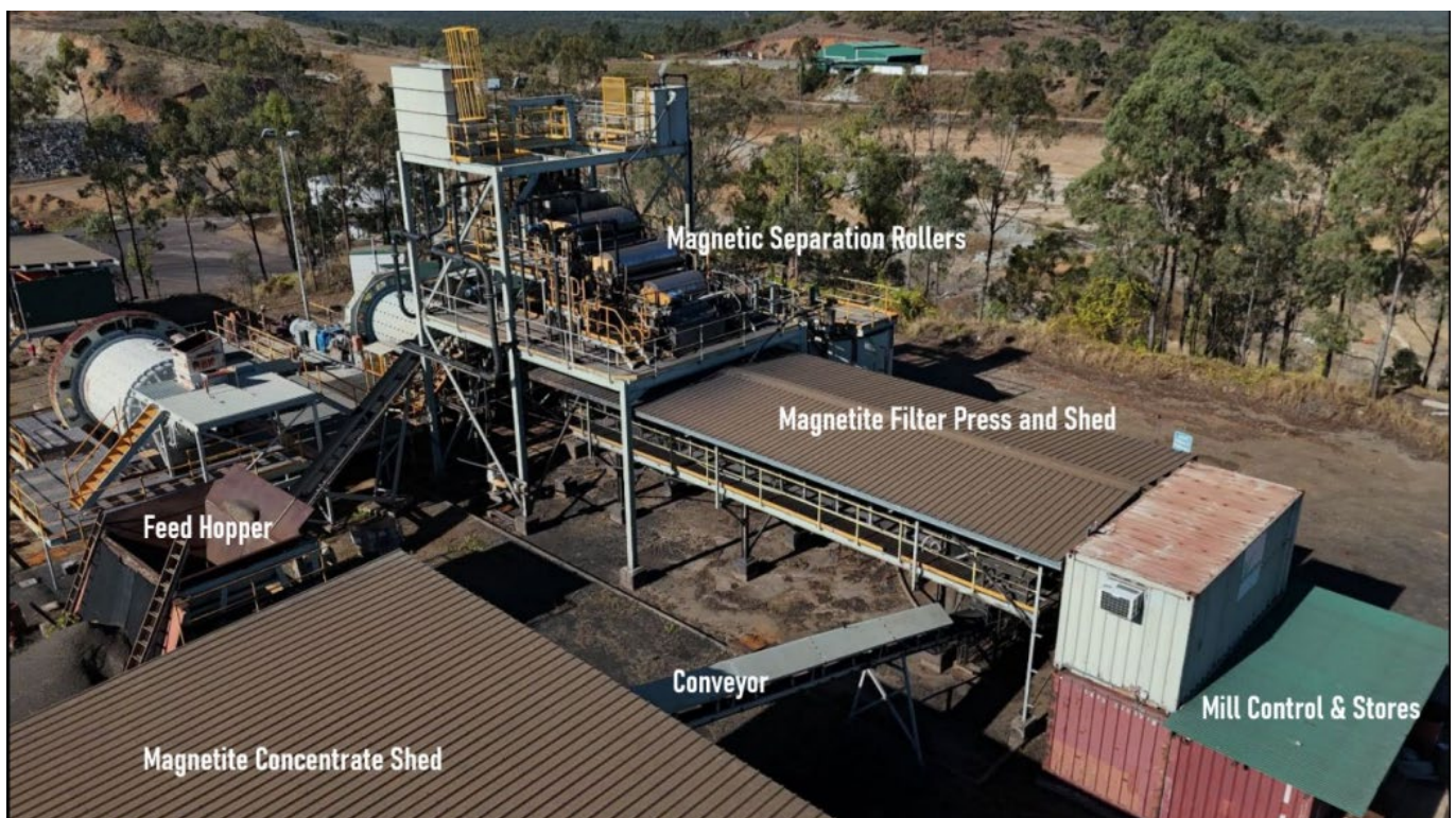
Figure 2 from ASX 8/9/26: Mt Moss Mill with all magnetite-related plant on July 13, 2026.
