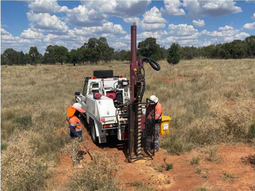
Figure 3 - Talisman Auger Drill Rig drilling on EL8571
