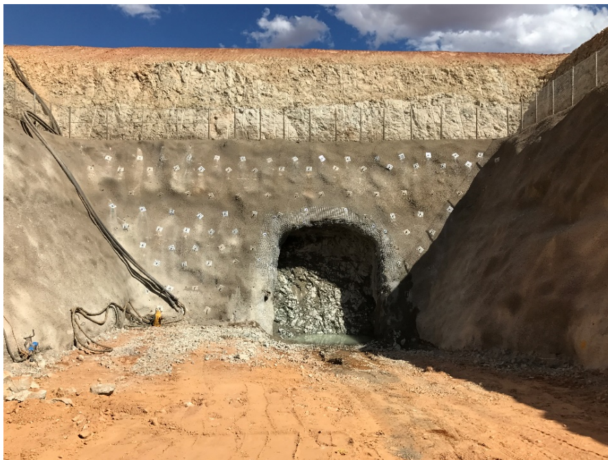
Figure 1: Monty Project – Bogged out first portal cut
