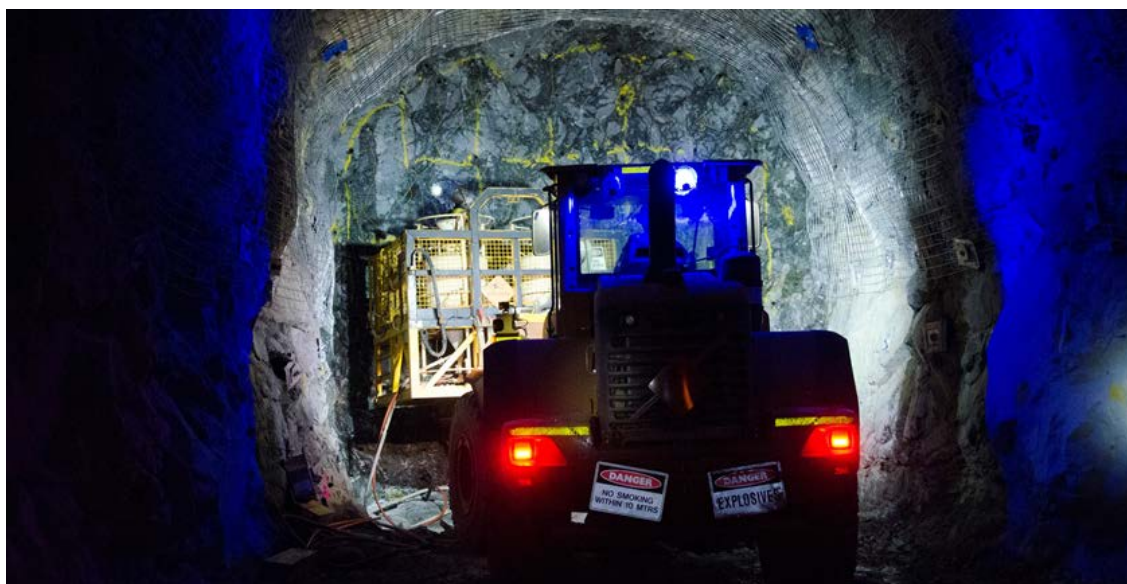
Figure 4: Monty Project: charging of the decline face, December 2017
