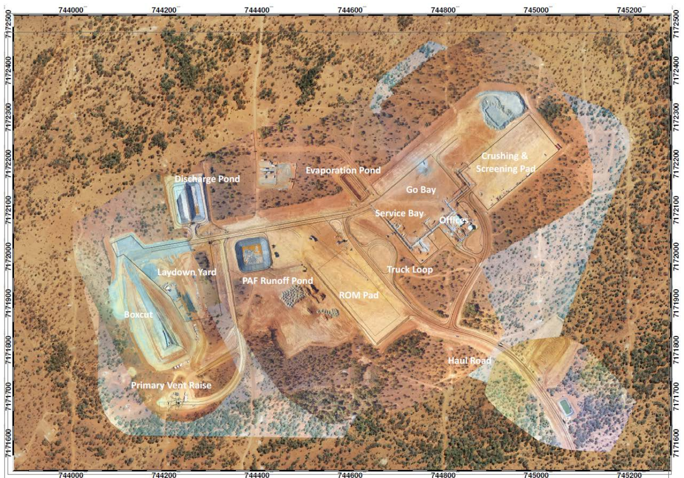
Figure 1: Monty Project: surface infrastructure layout and progress, December 2017
