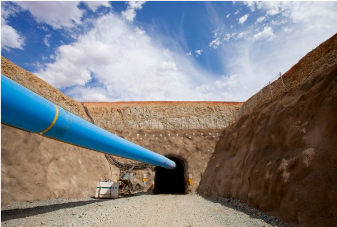
Figure 2: Monty Project: completed mine portal, December 2017
