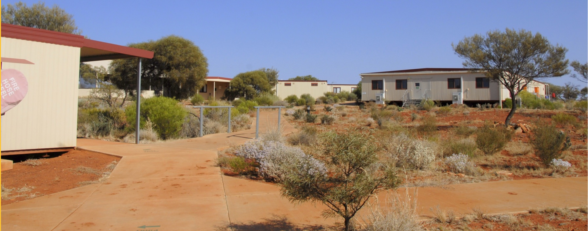
Sinclair Nickel Project – +200-person Accommodation Village
