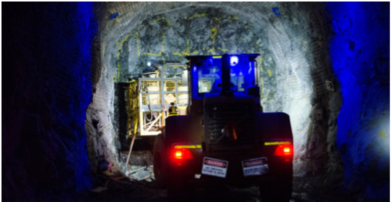
Figure 4: Monty Cu-Au Project: charging of the decline face, December 2017.
