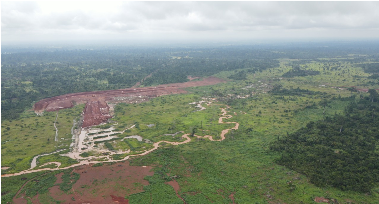
Figure 6: Water dam and diversion channel works
