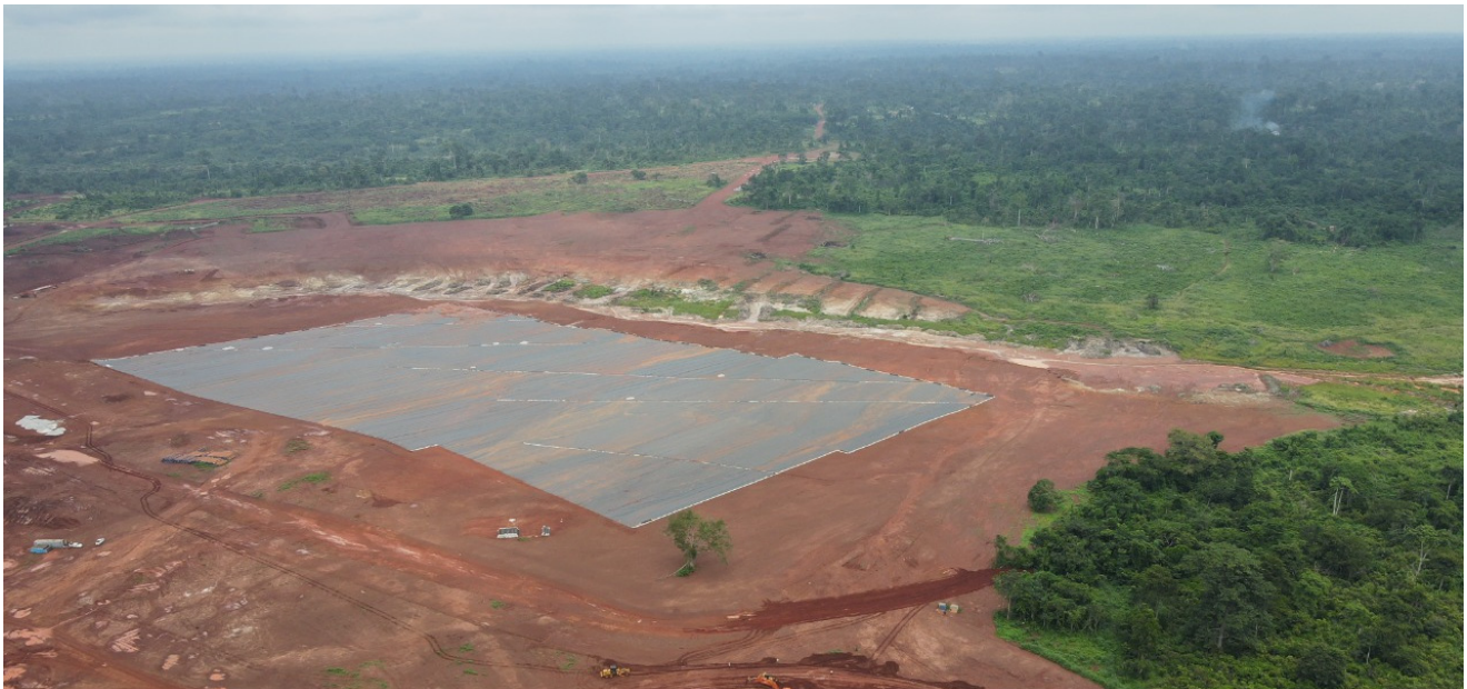
Figure 3: TSF - HDPE lining
