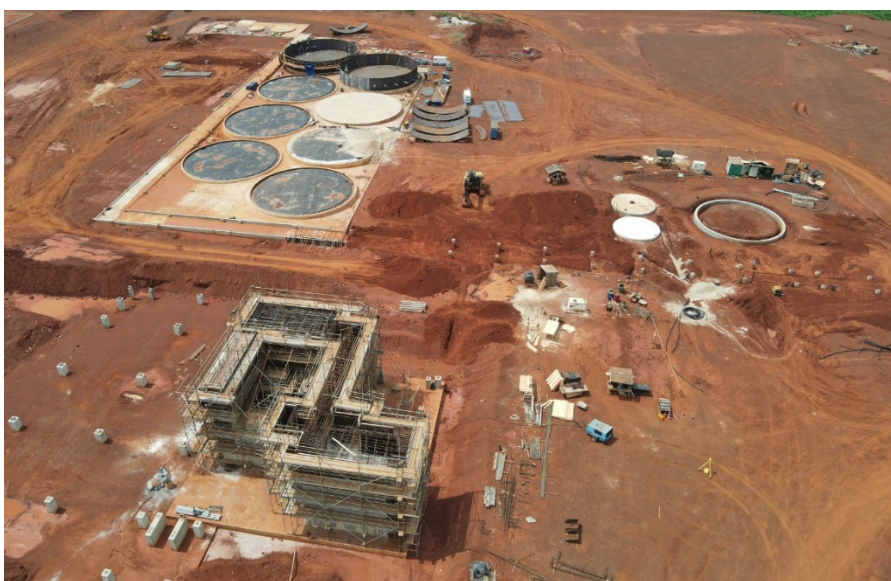
Figure 1: Overview showing Abujar's SAG Mill foundations and the first CIL tanks being erected (6 June 2022)
