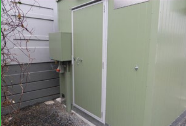
Zonecool™ shelter in use on site.
