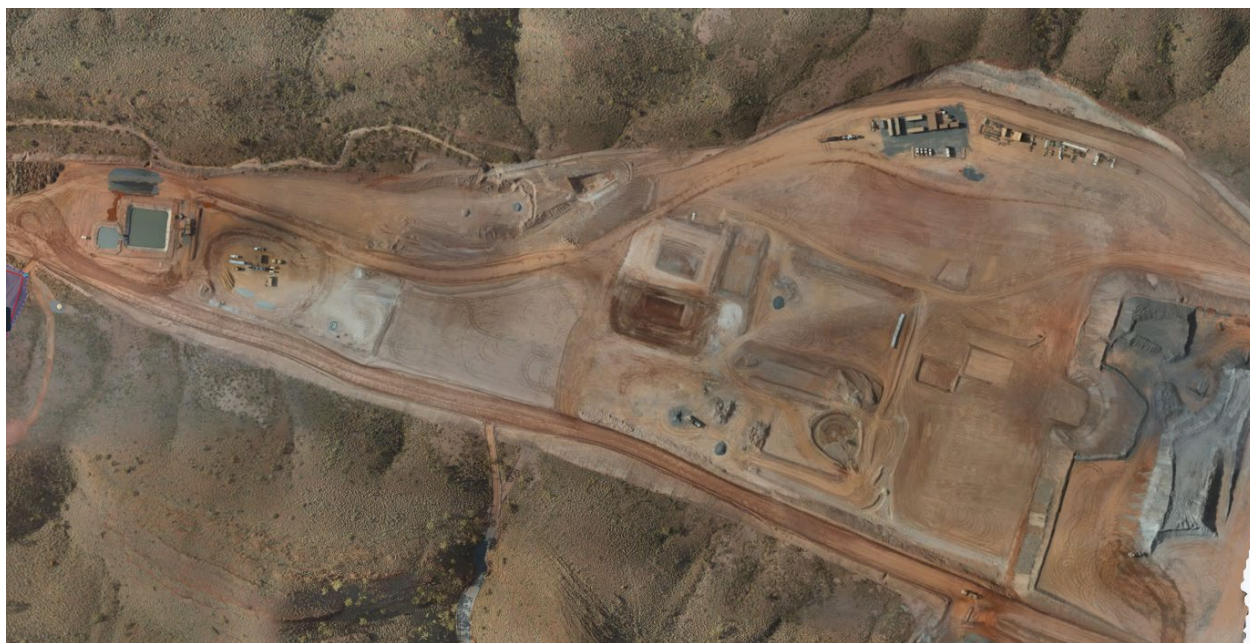
Figure 6: Yitirrti Mine plant site surface works September-26.
