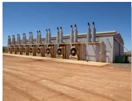
Gas/diesel power Infrastructure (KPS* gensets)
