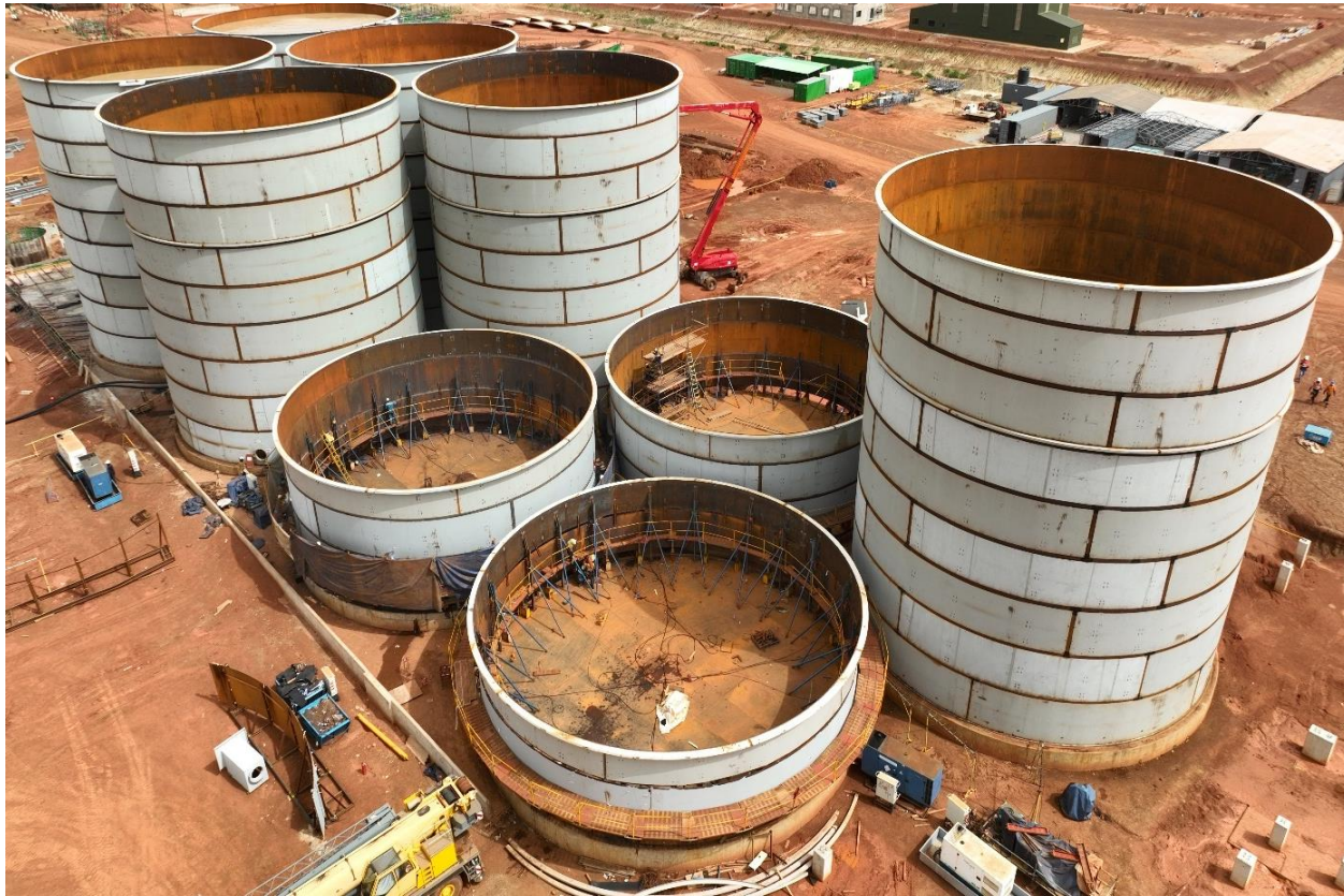
Kiaka Plant Construction: CIL tank fabrication and mills area & Bondek Base installation
