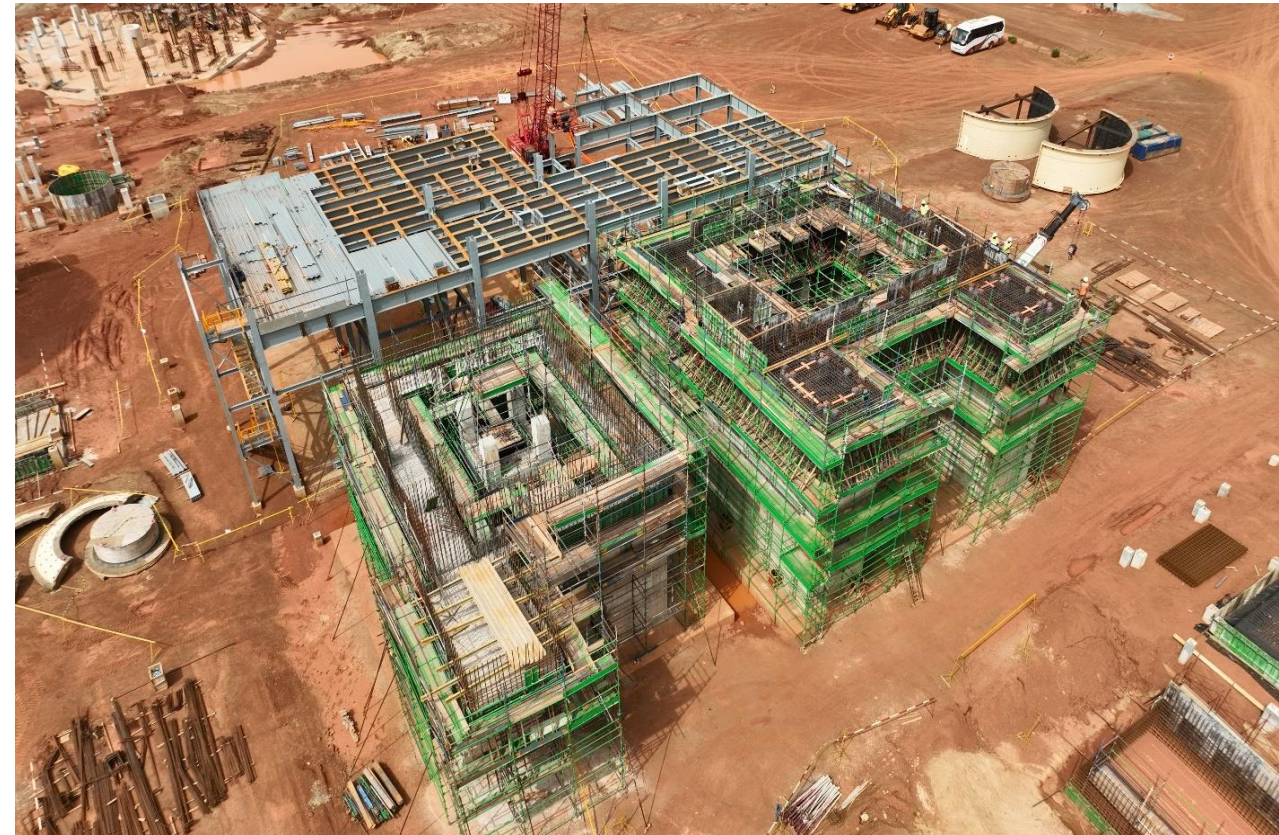
Kiaka Plant Construction: CIL tank fabrication and mills area & Bondek Base installation
