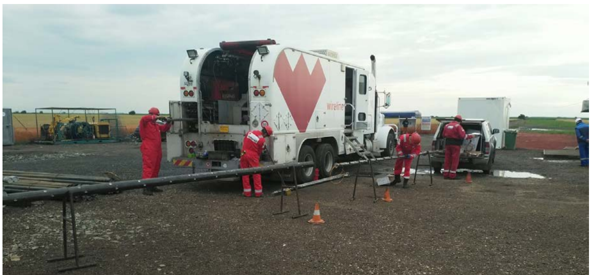
Preparation of perforation equipment prior to running into IMIC-1 well
