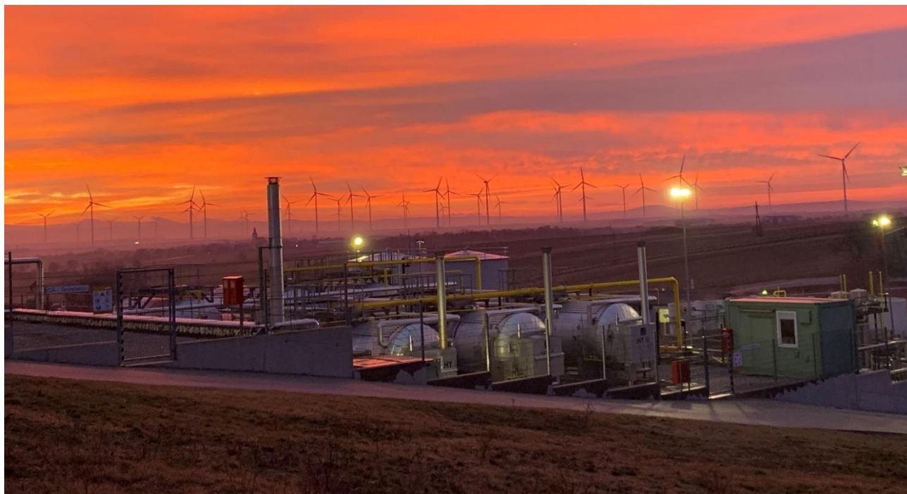
Figure 4: Photograph showing Gaiselberg and Zistersdorf infrastructure proximity to large wind farms capable of generating hydrogen.
