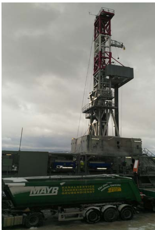
Drilling operations at Anshof-2 with the RED E-202 drilling rig.
