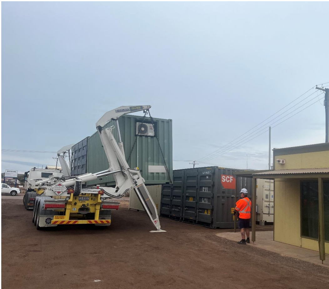
Delivery of modularised FRT pilot plant at Alligator's office/warehouse premises, Whyalla.
