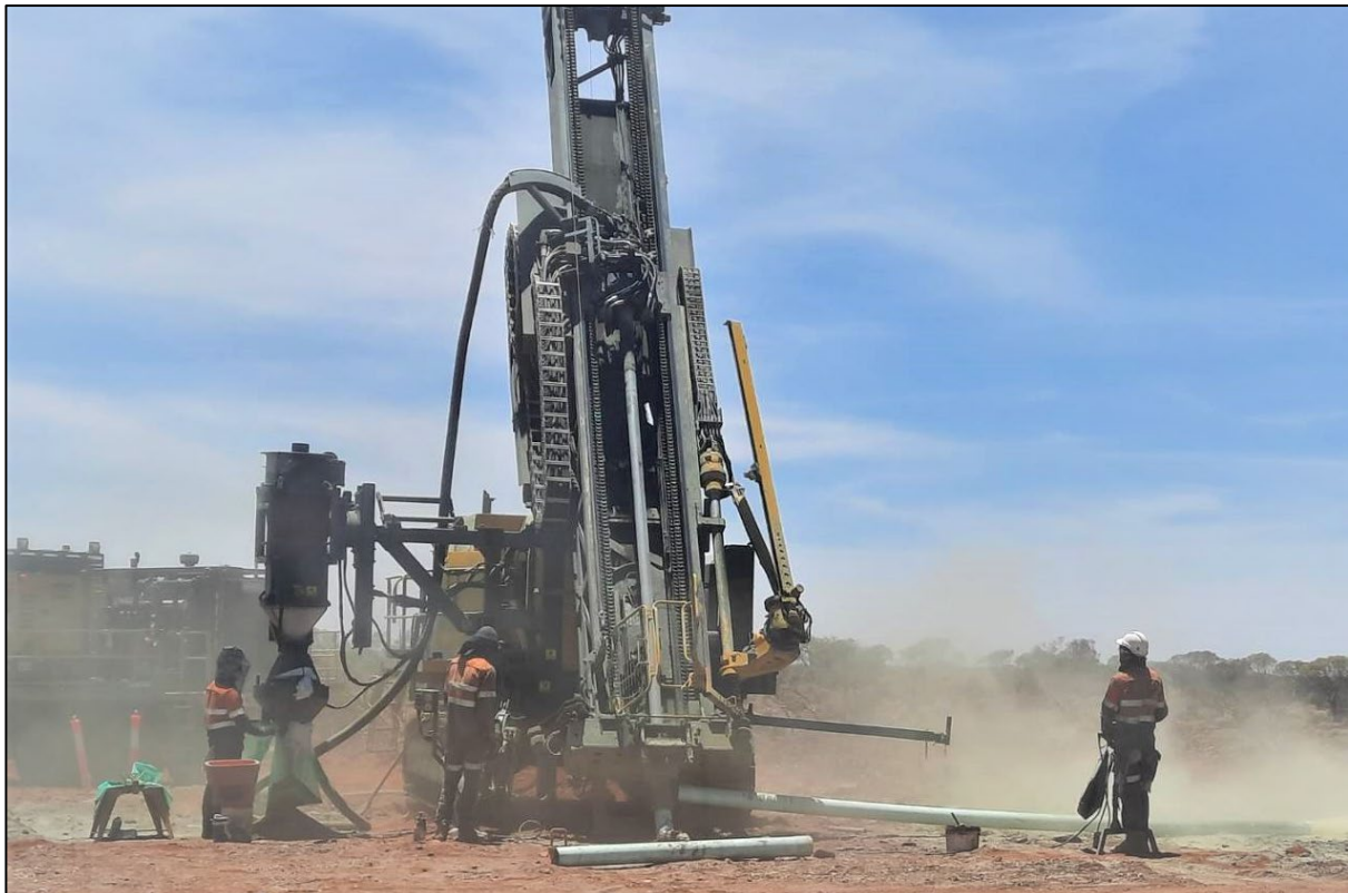
Figure 1. RC rig operating at Niobe.
