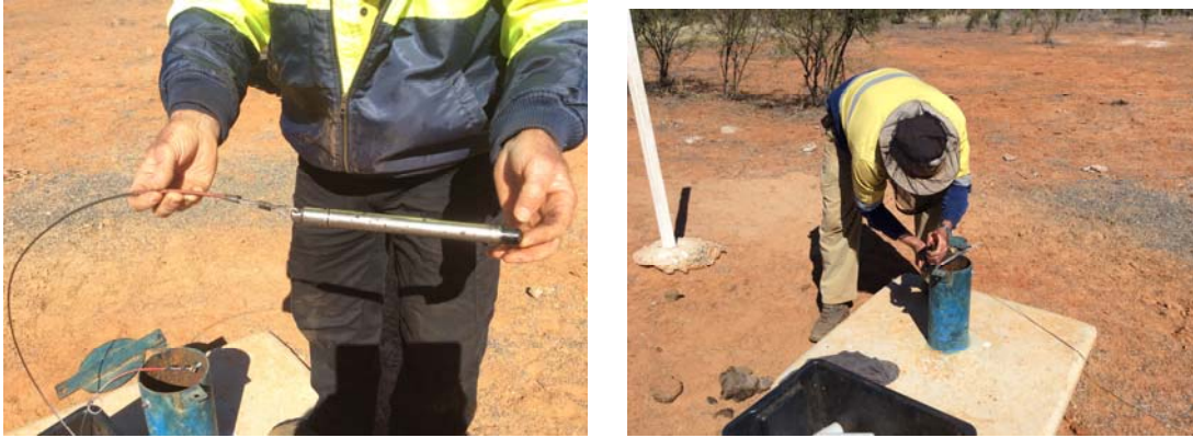
Installing dataloggers to continuously record groundwater data
