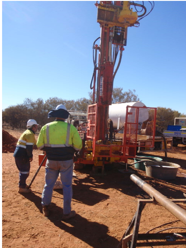
Geotechnical drillers completing Standard Penetration Test
