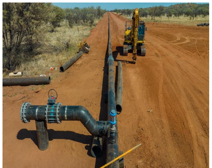
Figure 4: Water distribution pipe installation
