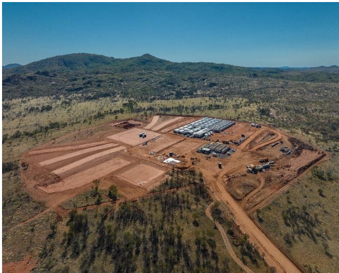
Figure 1: Aerial view of early works at Nolans Project
