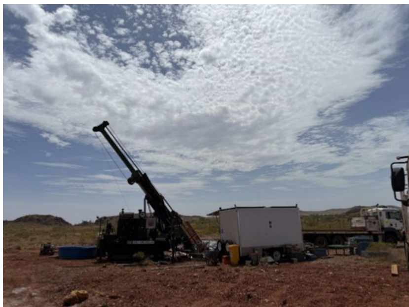
Figure 1: Diamond drilling underway at Titan East.
