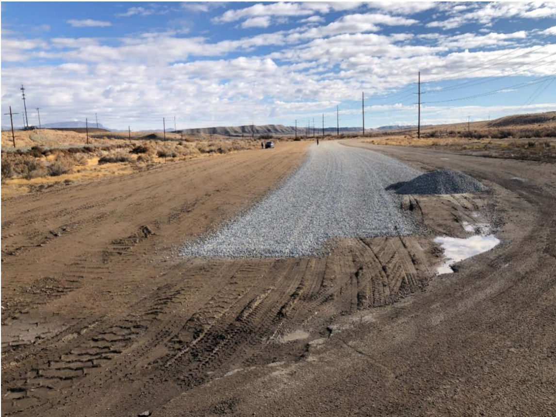
Figure 1: The base of the Demonstration Plant under construction at Green River.
