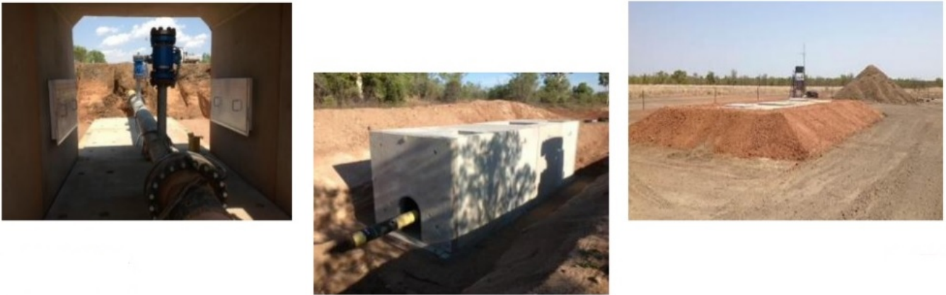
Figure 9: Century Mine underground slurry pipeline infrastructure
