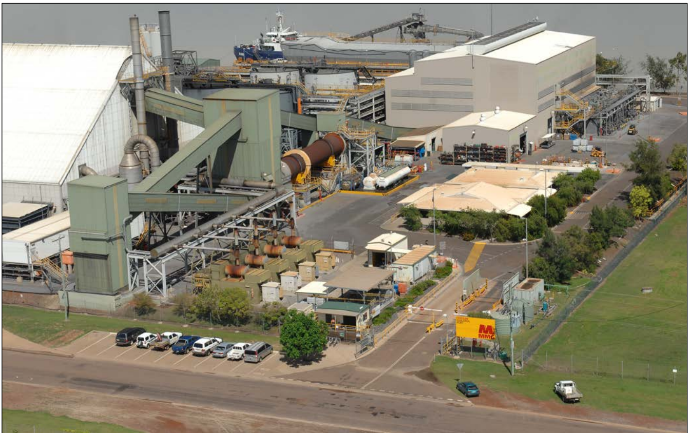
Figure 6: Karumba Port Facility
