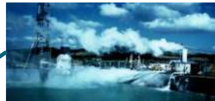
Pilot Plant Testing (C1 well, 1981-82)
