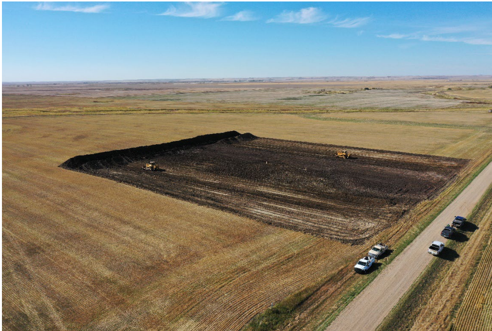
Figure 2: Construction of Pad #3
