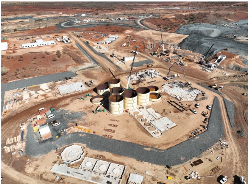
Figure 4: Construction progress at the Bellevue processing facility as at 19 February 2023
