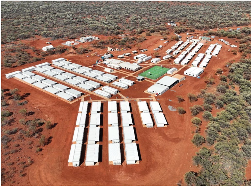
Figure 3: Bellevue's 343-person camp completed and commissioned during the December 2022 quarter
