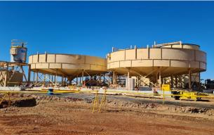
**Figure 7:** Construction progress on site at the end of April 2023 with partially painted CIL tanks, structural steel work well advanced on the crushing and screening areas and fine ore bin construction commenced.
