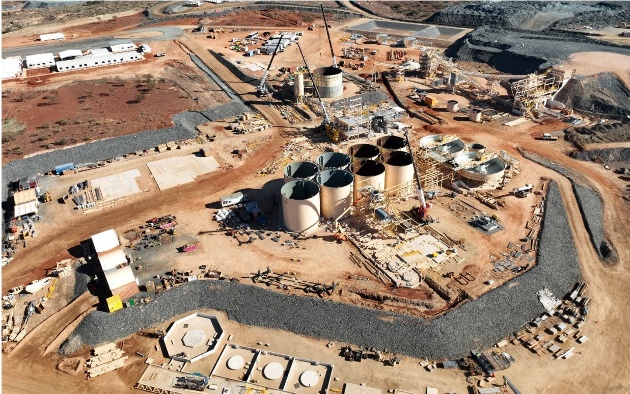
Figure 4: Processing Plant construction progress 21 May 2023.
