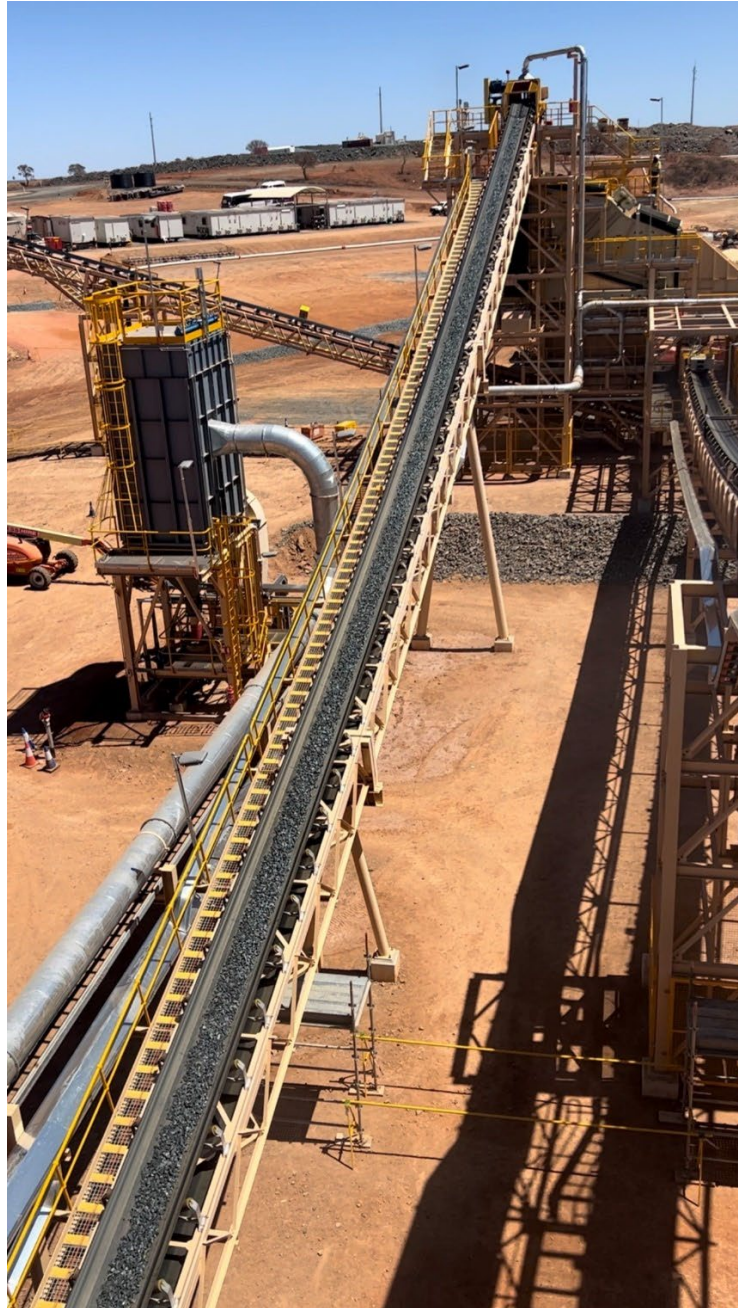
Figure 3: Crushing circuit commissioning has commenced with first material fed through circuit.
