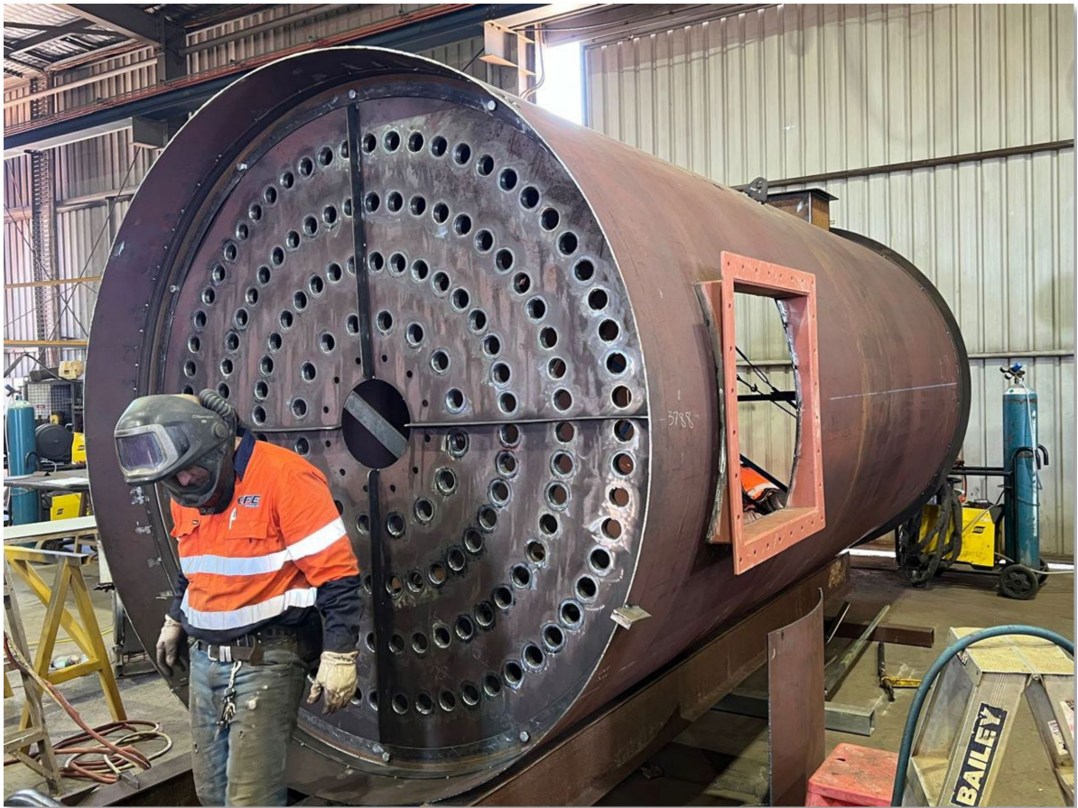
Figure 17: CIC tank 1 under construction for delivery to site
