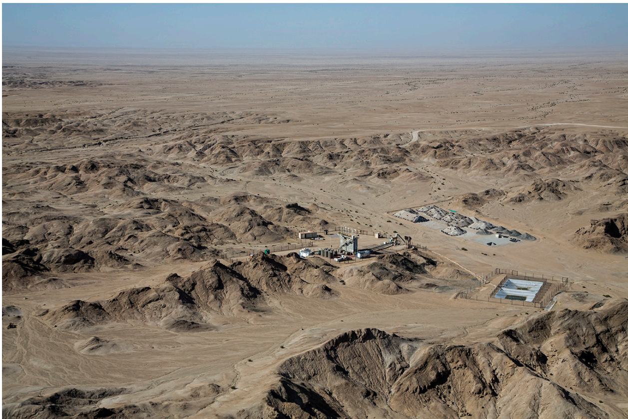
Etango Uranium Project, Namibia, showing Etango Heap Leach Demonstration Plant
