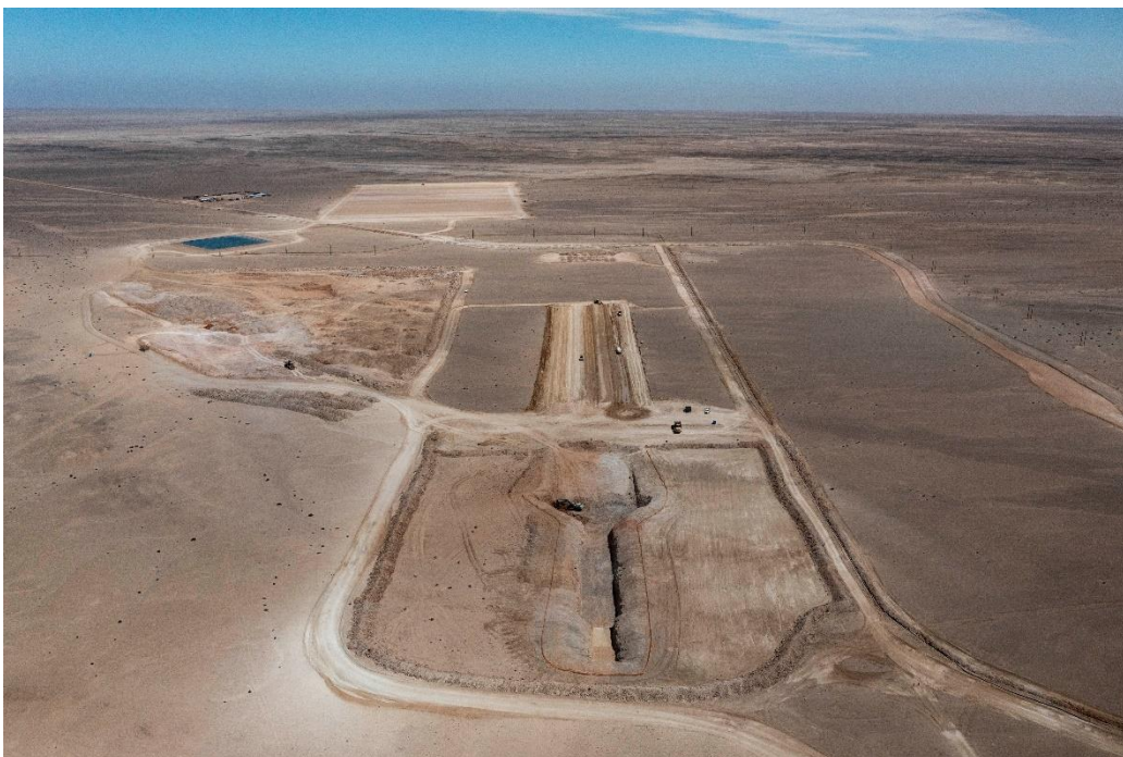
Figure 1: Significant progress continues on bulk earthworks at Etango, a key enabler of future construction and development activities. The primary crusher has been fully excavated and its dimensions confirmed, while work advances on the permanent road and conveyor belt line to the secondary and tertiary crushing areas.
