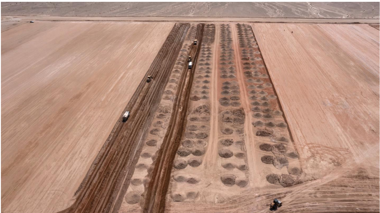
Figure 1: Heap leach earthworks continue to advance strongly.
